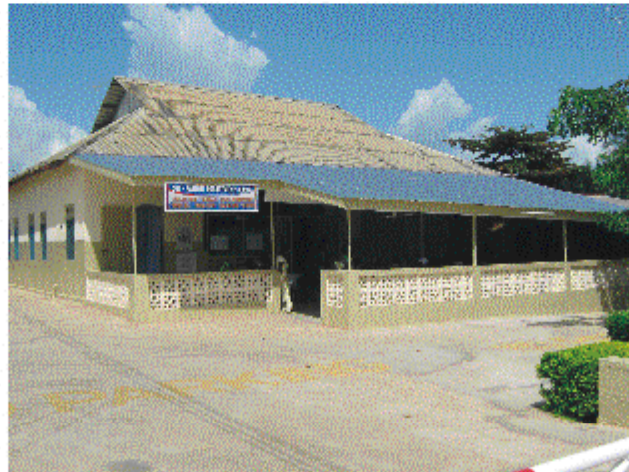
P DC Rehabilitated old OPD waiting area
