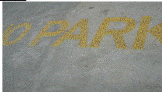
P DC Concreted floor
